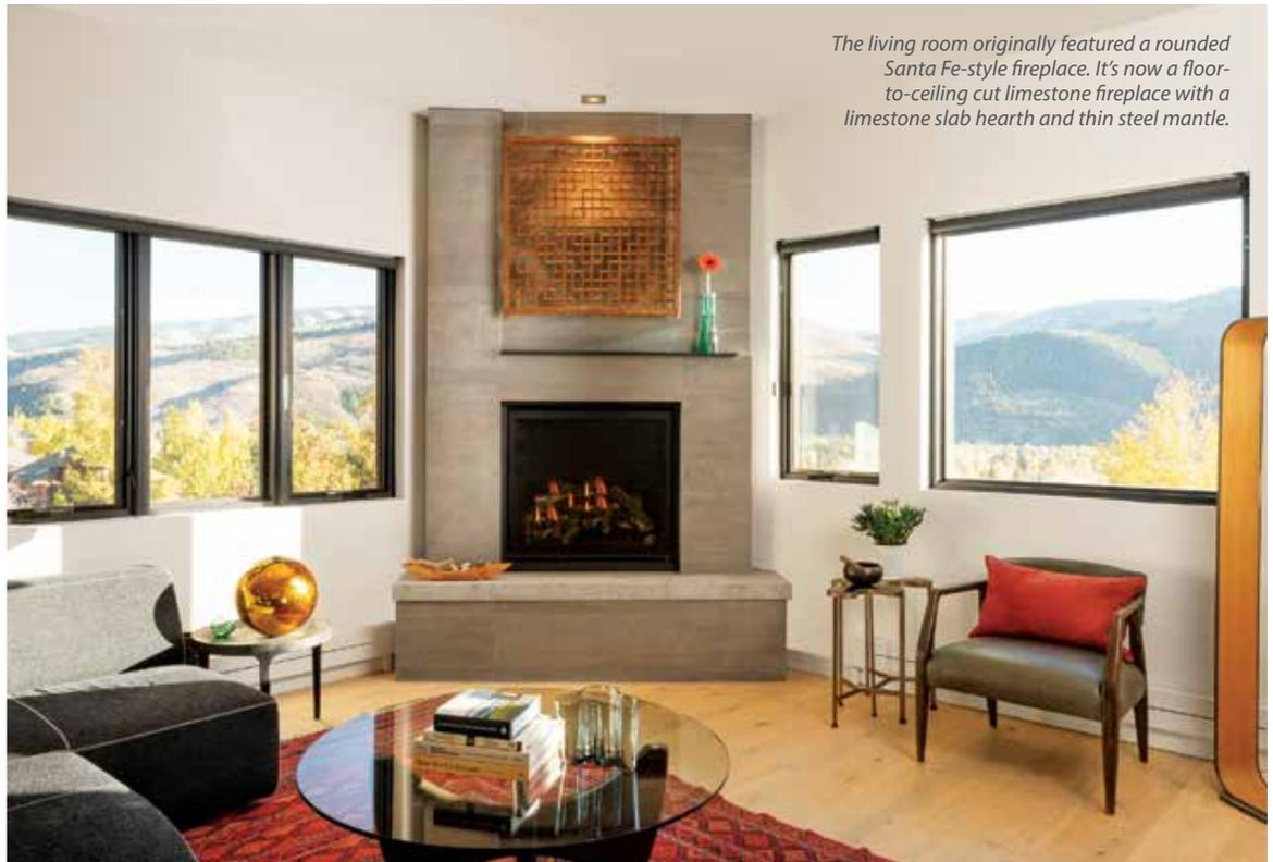
*The living room originally featured a rounded Santa Fe-style fireplace. It's now a floor-to-ceiling cut limestone fireplace with a limestone slab hearth and thin steel mantle.*
